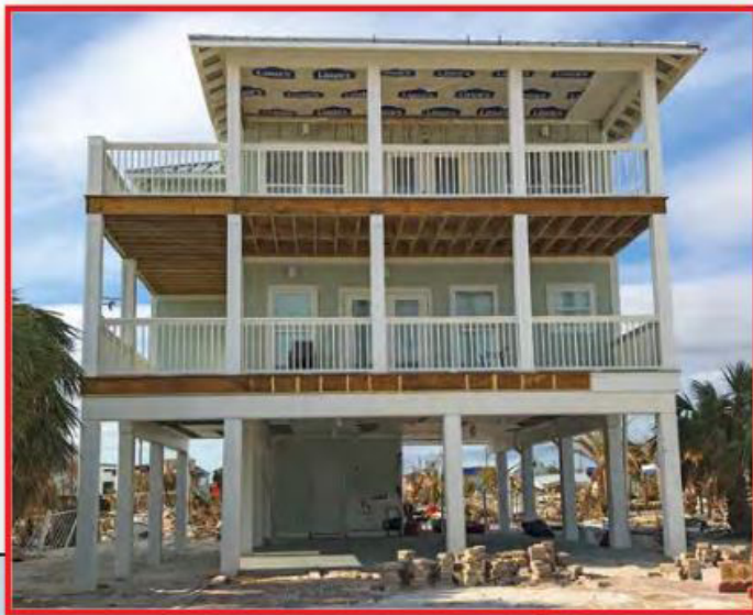
Exhibit 11 Representative adjacent single-family dwellings elevated on concrete piles that survived the hurricane (Mexico Beach; unshaded Zone X)
