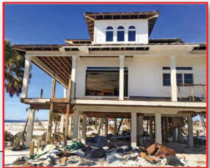
Exhibit 11 Representative adjacent single-family dwellings elevated on concrete piles that survived the hurricane (Mexico Beach; unshaded Zone X)
