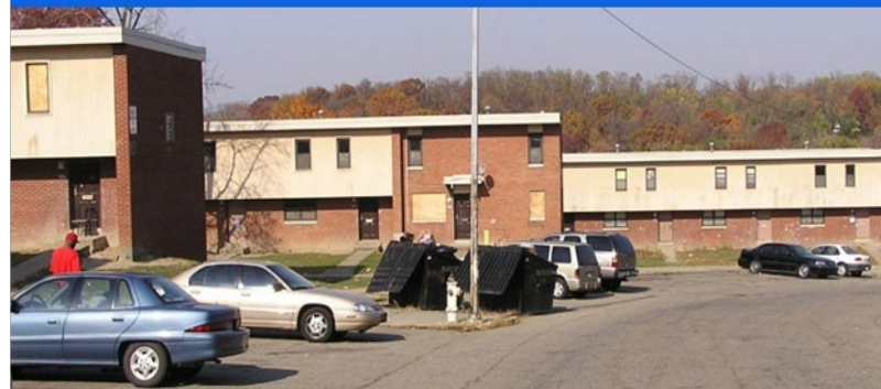
Garfield Heights – Before Redevelopment
