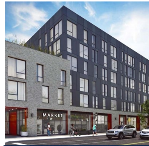
Roosevelt Square Phase 3B, a 207-unit development with 75 Faircloth-to-RAD units in Chicago, IL
