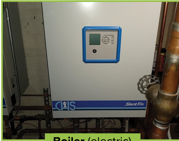
Boiler (electric)
