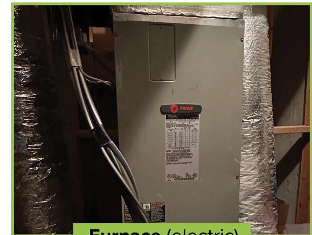
Furnace (electric)
