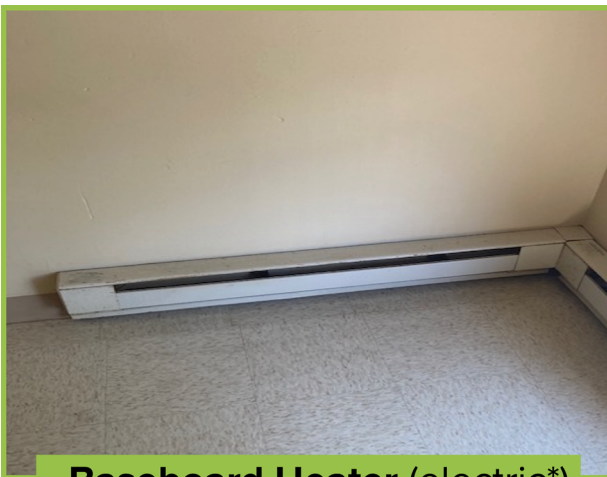
Baseboard Heater (electric*)
