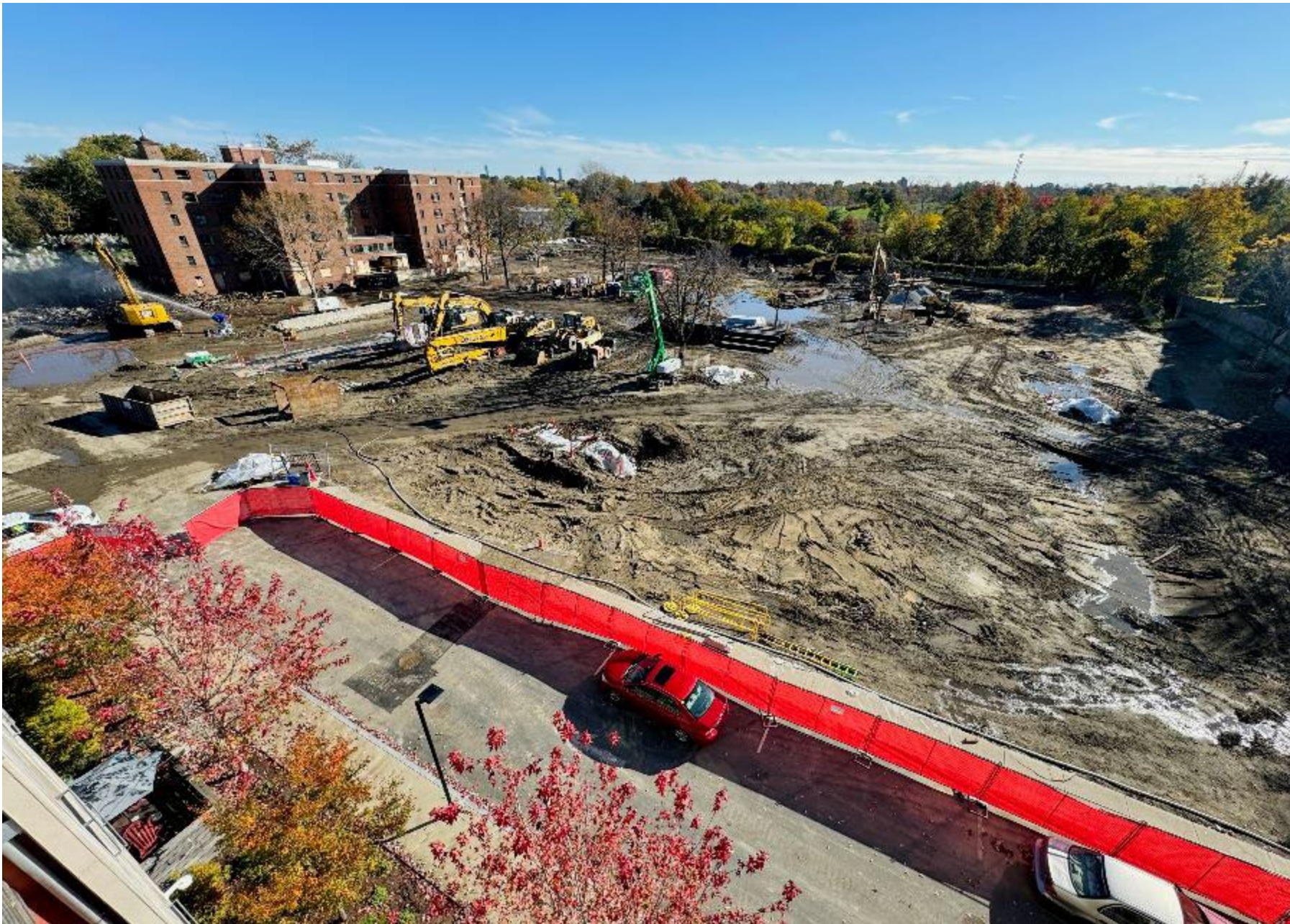
At Jefferson Park Federal, demolition is complete
