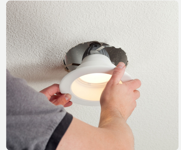
Installing LED retrofit bulb into single-family home
