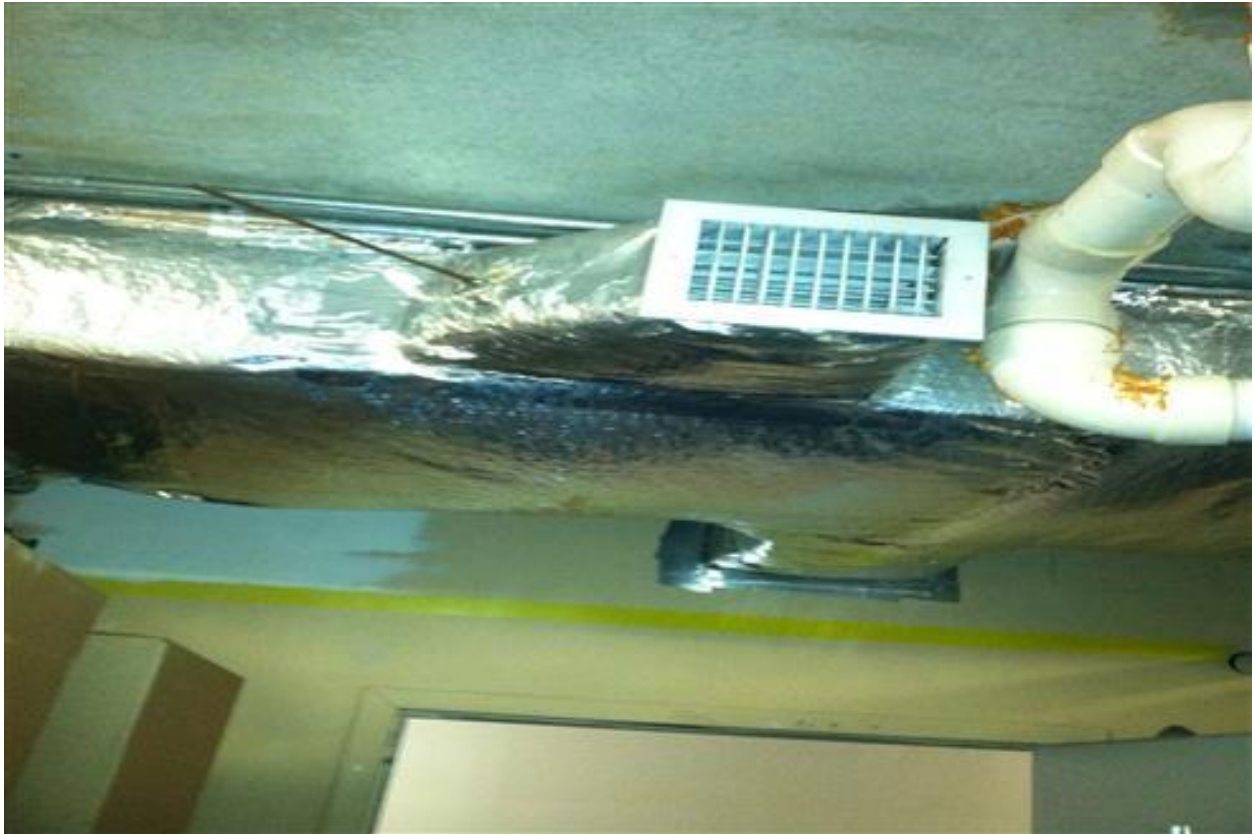
19 - FIBERGLASS-INSULATED DUCTS
