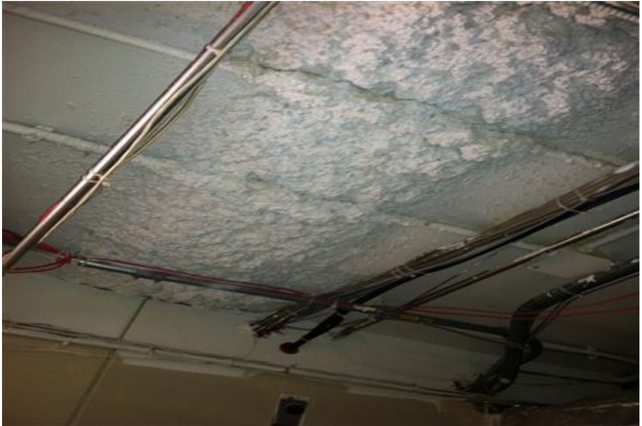
11 - SPRAY-ON FIREPROOFING ON BASEMENT STEEL BEAM
