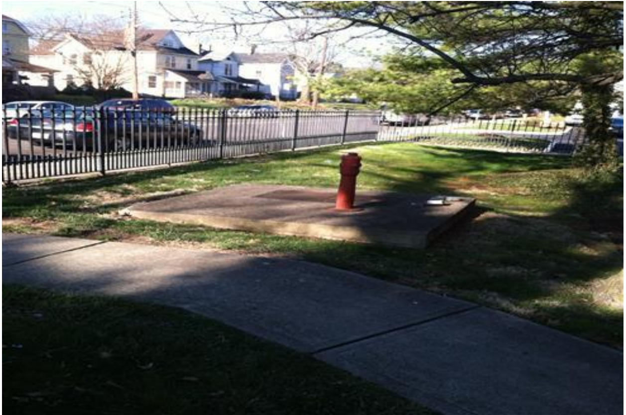
43 - PUBLIC WATER SUPPLY ON-SITE
