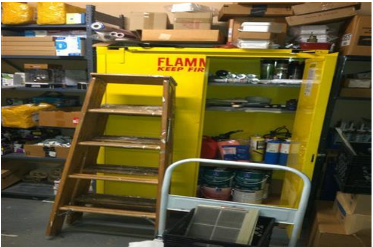
24 - FLAMMABLES STORAGE CABINET
