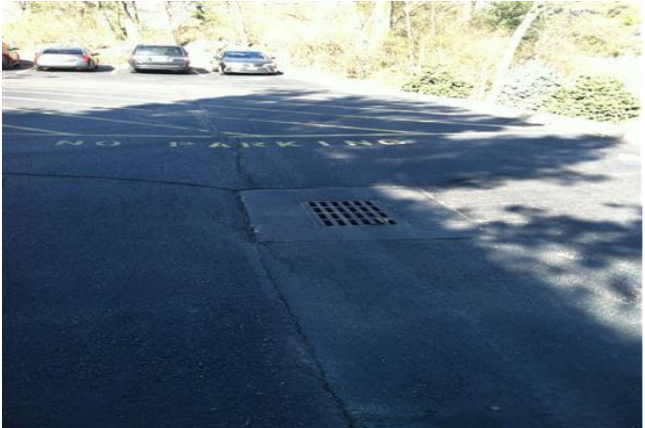
45 - PARKING LOT STORM WATER INLET
