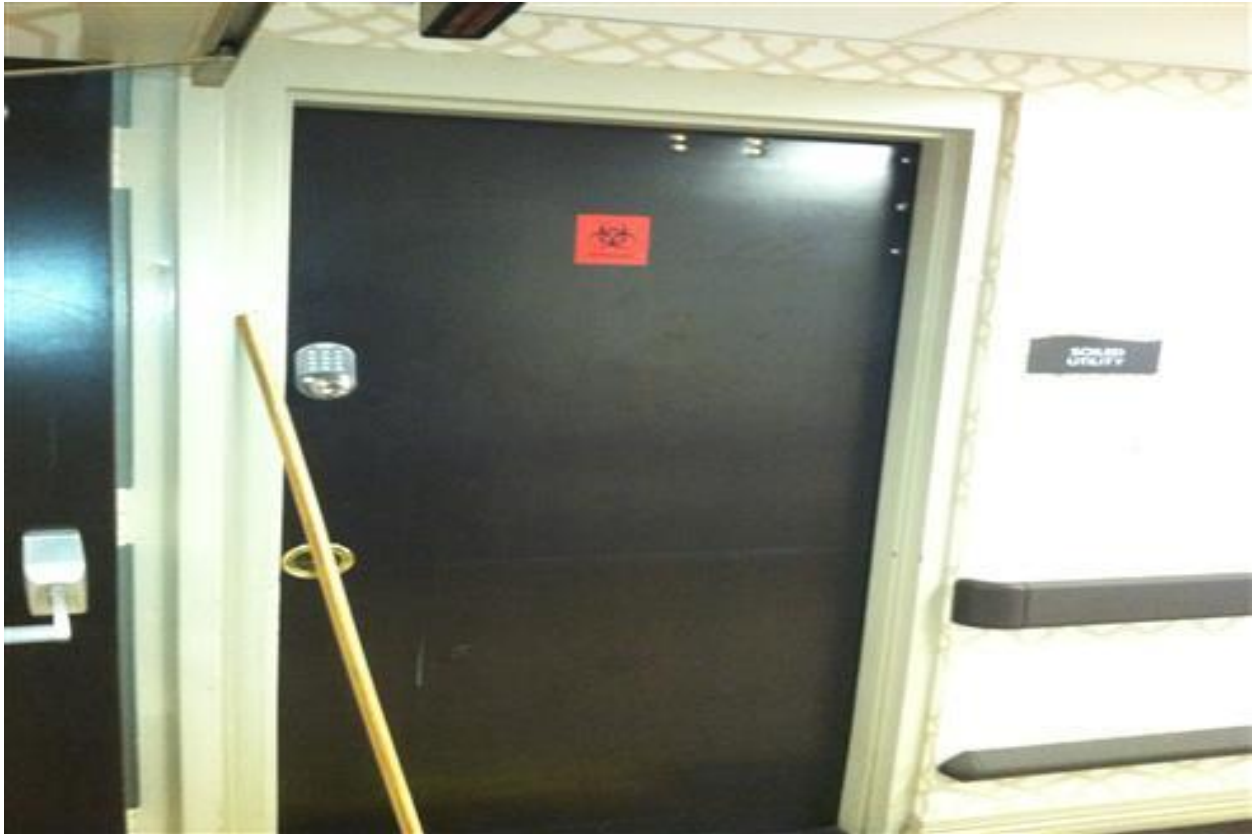
29 - BIOHAZARD STORAGE CLOSET
