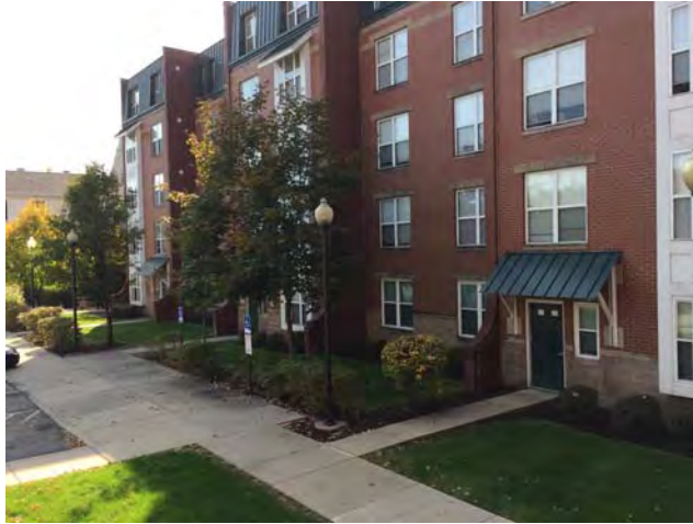
View of rear portion of main apartment building
