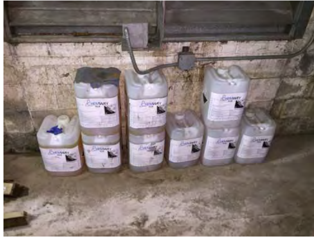
View of glycol storage in utility room of main apartment building
