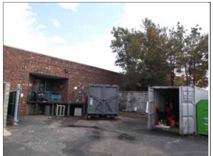
18. View of Trash Compactor and Container Storage
