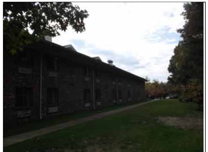
4. View of Rear Elevation
