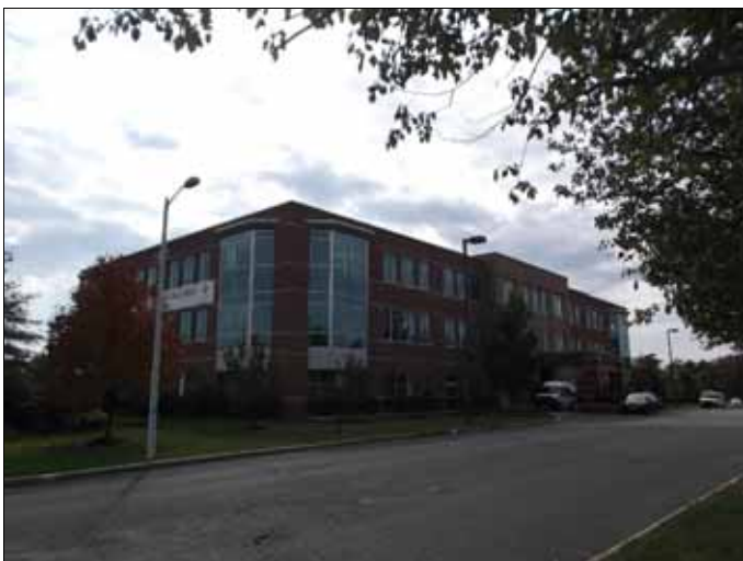
23. View of South adjacent commercial
