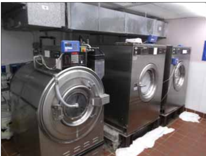
11. View Laundry Room
