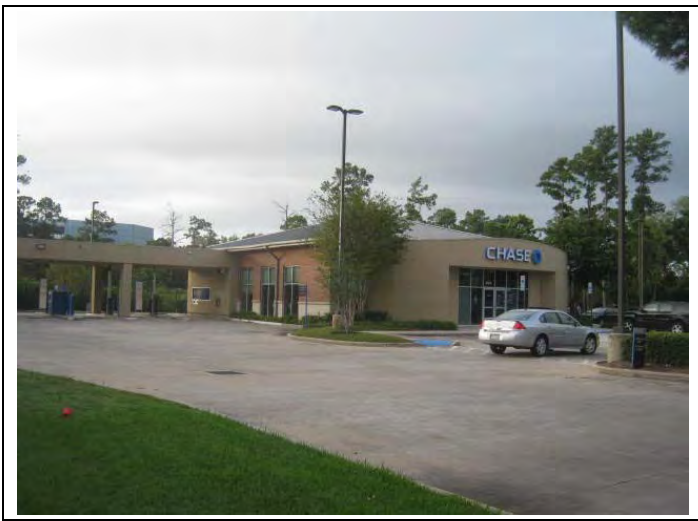
1. View of the Chase Bank facility adjoining to the east.
