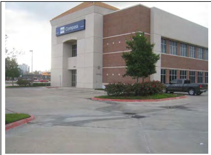
5. View of the Compass Bank adjoining to the east.
