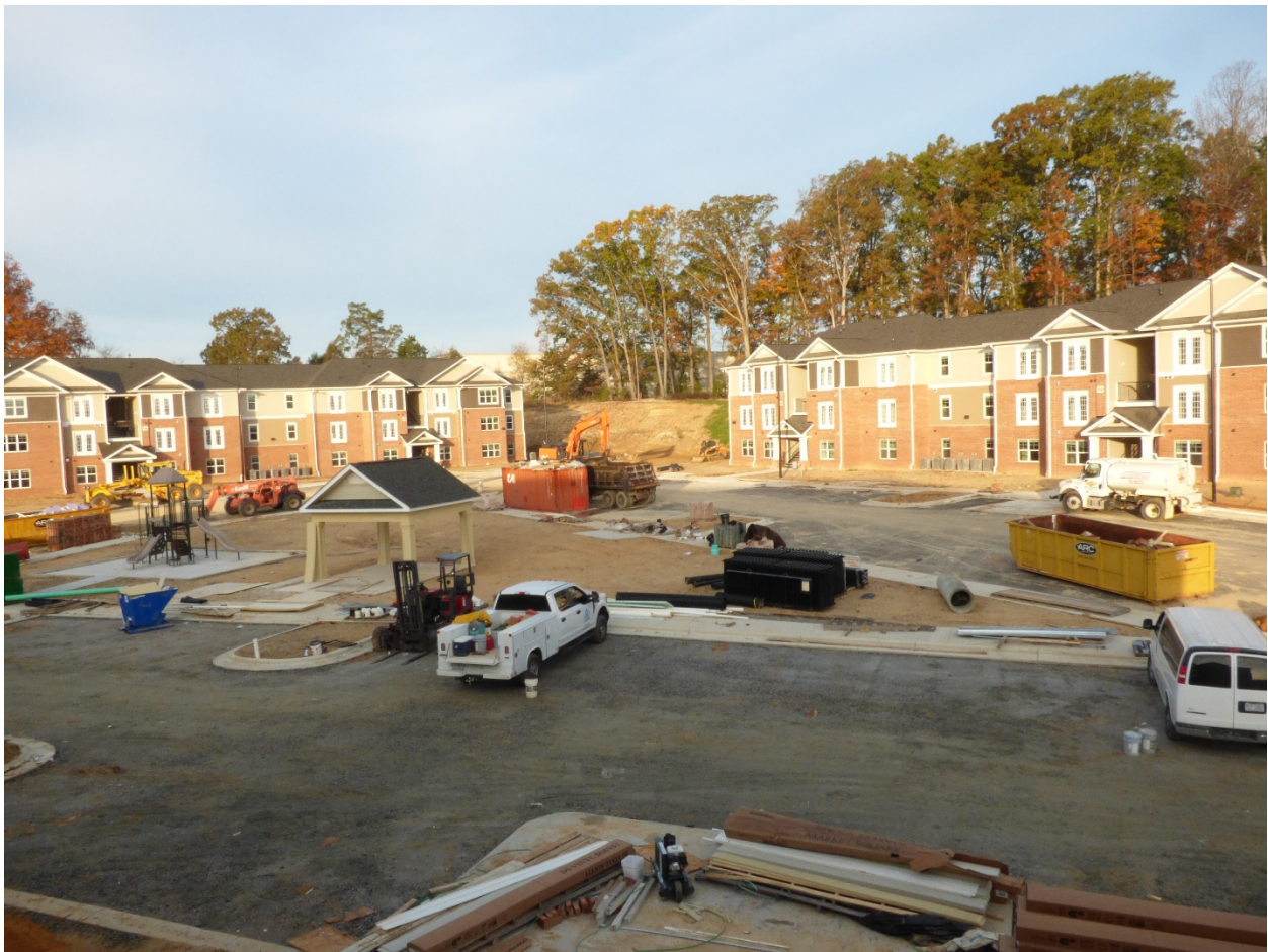
Avondale Trace Apartments (Under Construction)
