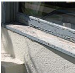
FIGURE 5.4a Peeling paint
