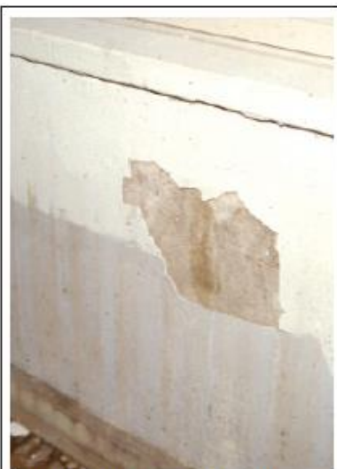
FIGURE 5.5 Baseboard showing a de minimis amount of deteriorated paint.
