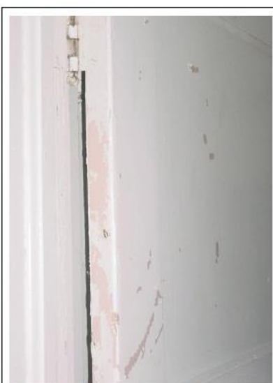
FIGURE 5.7 Impact surface on door and frame.
