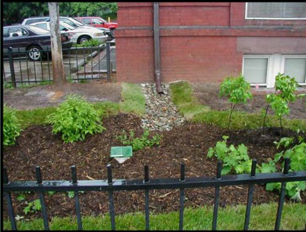
Disconnected downspout and bioretention cell, Capital Hill, Washington, DC. Photo courtesy of LID Center.
