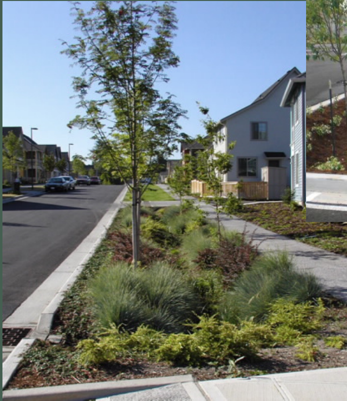
Permeable pavement and bioretention in Albuquerque, NM. Photo courtesy of AridLID.org.
