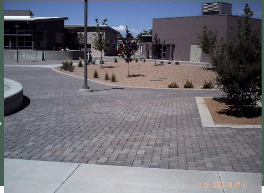
Bioretention Cell in El Monte, CA. Photo courtesy of Bill DePoto.
