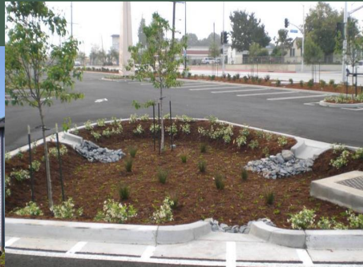
Bioretention Cell in El Monte, CA. Photo courtesy of Bill DePoto.
