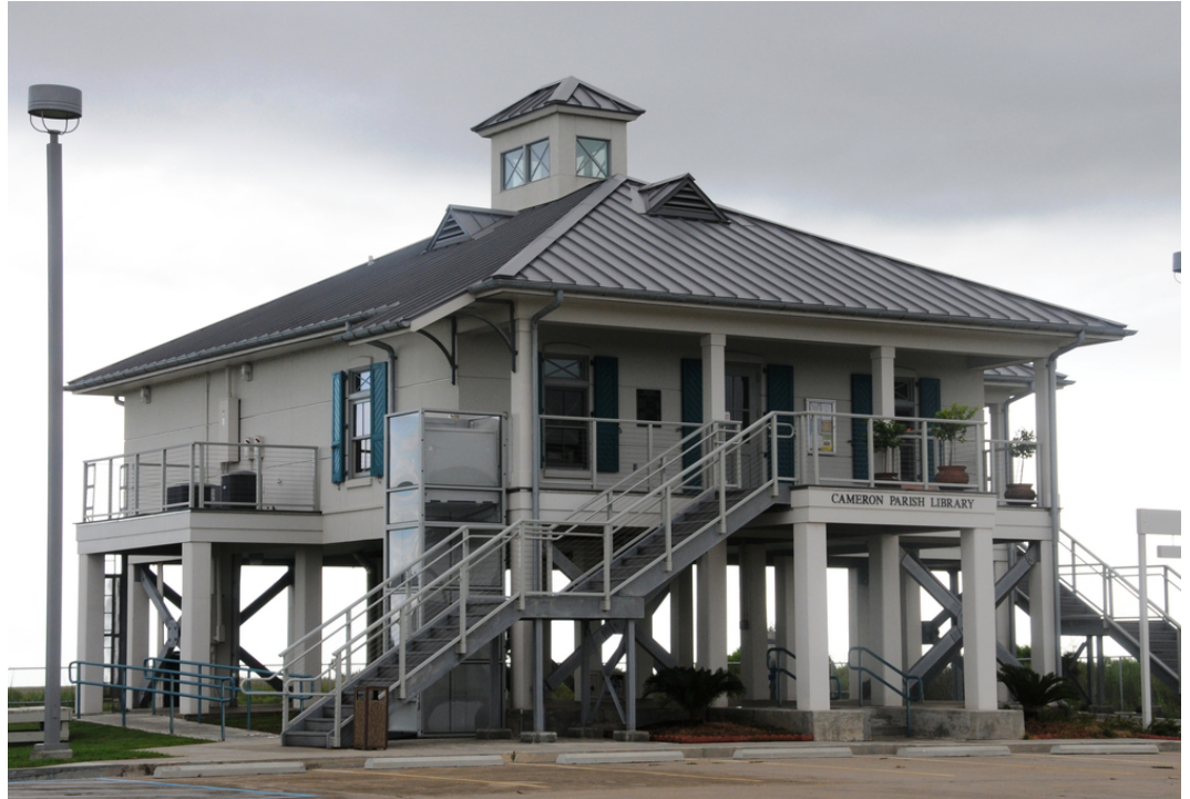
Johnson Bayou Branch Library Cameron Parish, LA, July 20, 2013 Source: FEMA News Photo / Lillie Long
