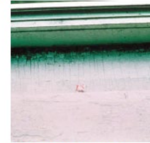
FIGURE 5.4b Alligatoring paint
