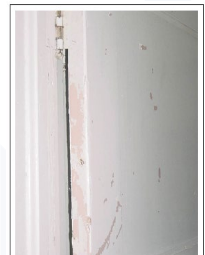
FIGURE 5.7 Impact surface on door and frame.
