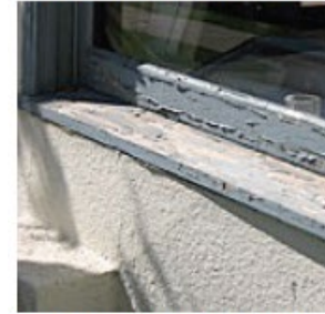
FIGURE 5.4a Peeling paint
