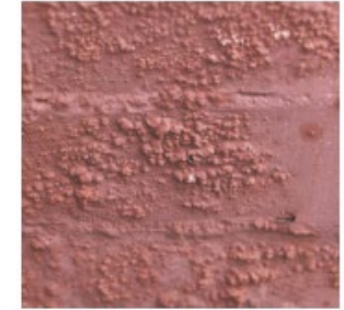
FIGURE 5.4c Blistering paint
