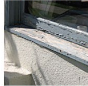
FIGURE 5.4a Peeling paint
