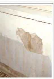
FIGURE 5.5 Baseboard showing a de minimis amount of deteriorated paint.
