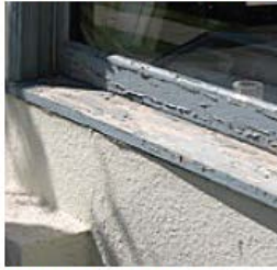
FIGURE 5.4a Peeling paint
