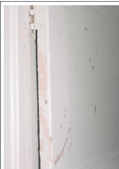
FIGURE 5.7 Impact surface on door and frame.
