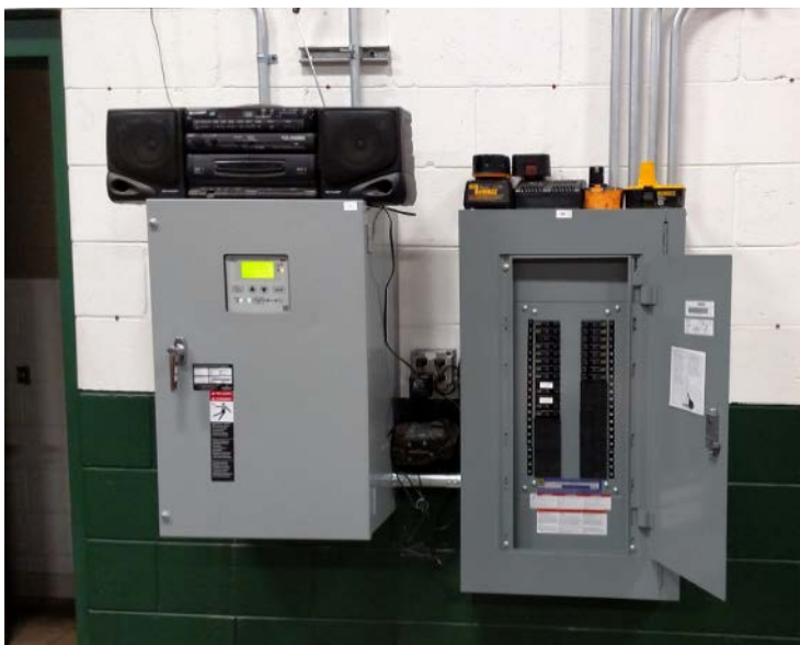
Left: Automatic Transfer Switch
