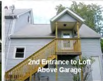
2nd Entrance to Loft Above Garage
