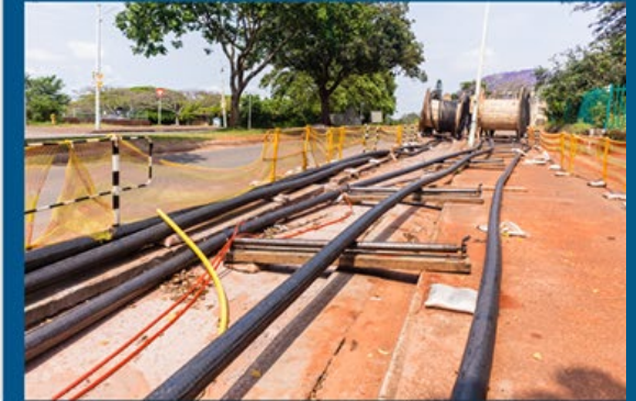
Installing underground electrical lines
